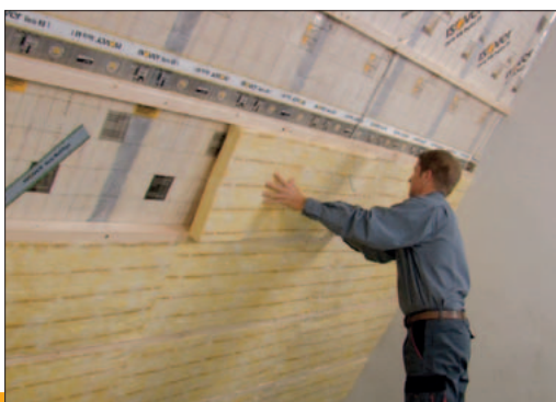
Example of product application ISOVER Multiplat 34 NT
