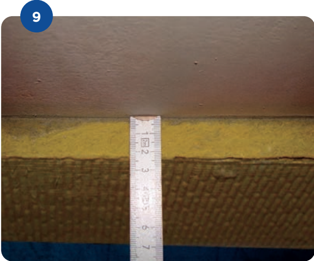
Check the system thickness, 20 mm slab, 3-4 mm layer of adhesive
