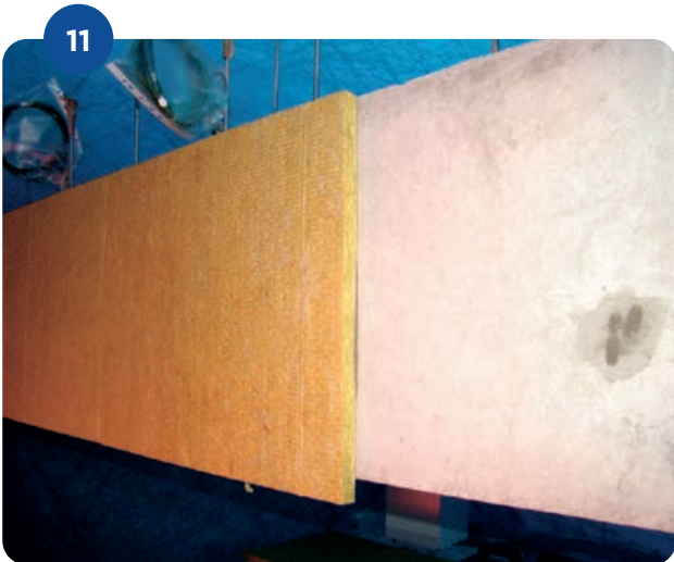
In case of a beam, the sides are glued first
