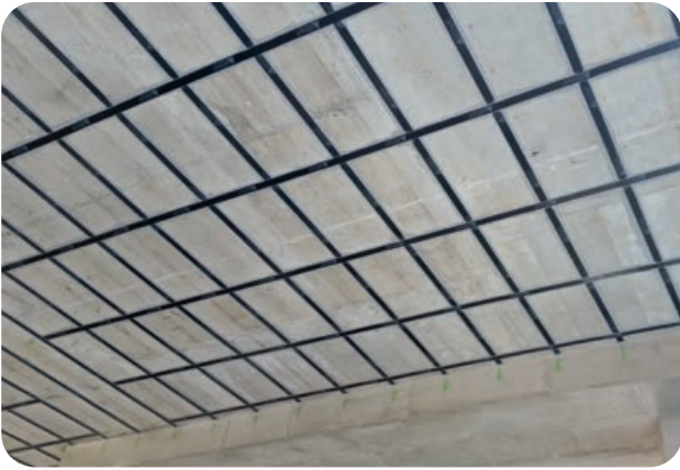
Fig. 17 Carbon fiber reinforced lamellas before fire protection
