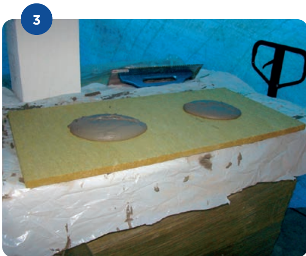
Apply an adequate amount of the adhesive on the slab
