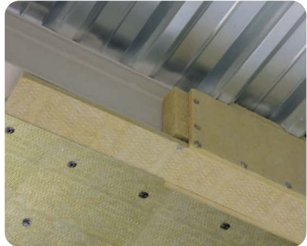
Fig. 15 The four side fire protection of a steel beam (using the Isover FireProtect® 150 slabs to backfill a trapezoidal profile)
