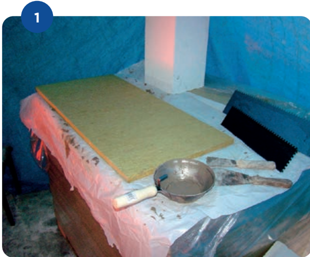
Inspect the slab and the tools used
