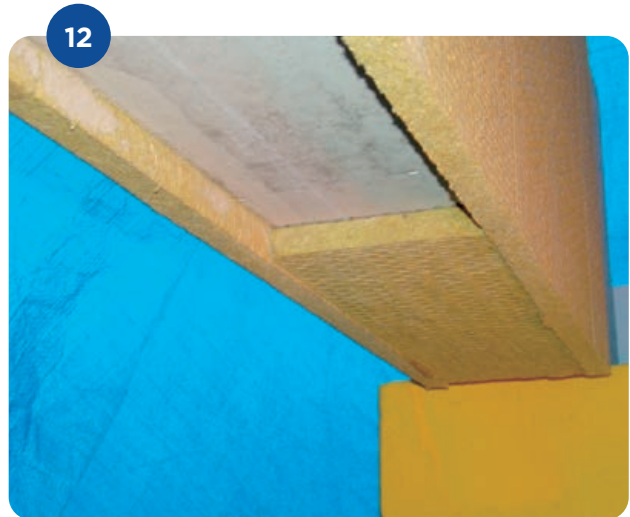
The flange is glued in the end
