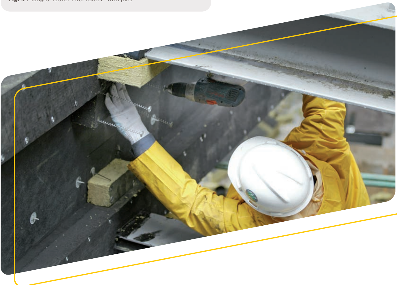
Fig. 4 Fixing of Isover FireProtect® with pins
