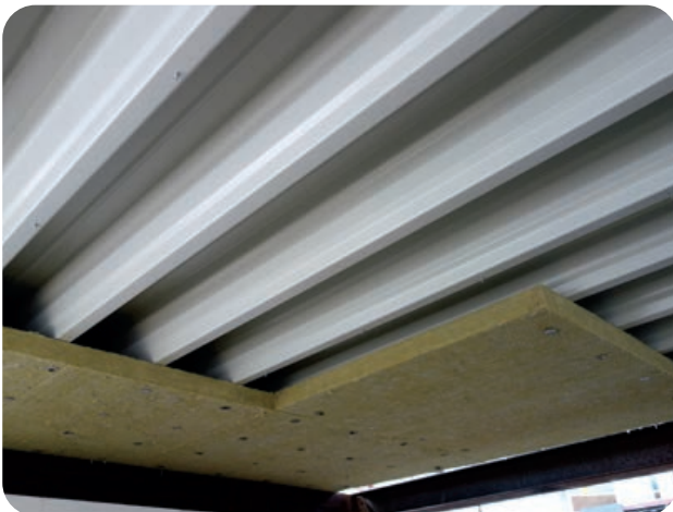
Fig. 10 System Isover FireProtect® for fire protection of corrugated steel is characterized by light weight and small height, but also a direct fixing to the corrugated steel without need of help of suspension construction
