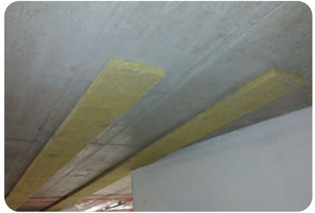
Fig. 18 Semifinished fire protective cladding ORDEXAL® KARBON ALB without final surface layer
