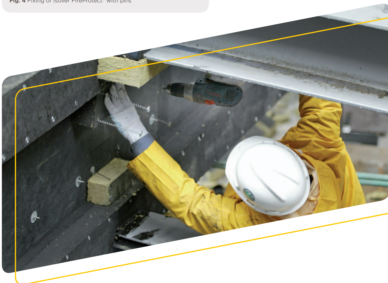
Fig. 4 Fixing of Isover FireProtect® with pins
