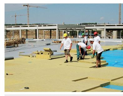
Fig. 1 - Example of Isover T-i application
