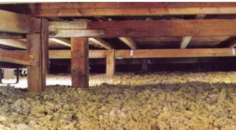
Fig. 5 - Blown insulation
