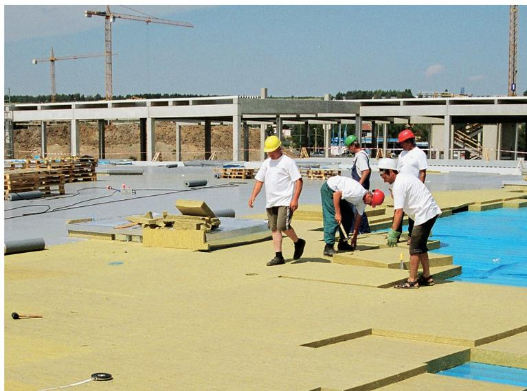
Fig. 1 - Example of Isover T-i application
