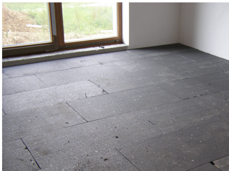
Fig. 1 - Example of Isover EPS Grey 100 application
