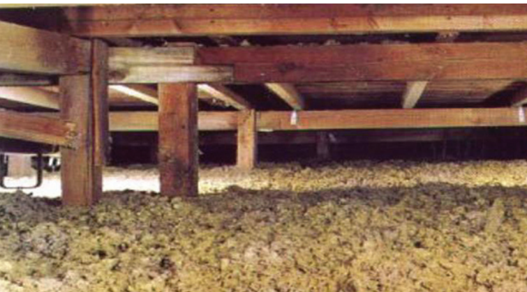
Fig. 5 - Blown insulation
