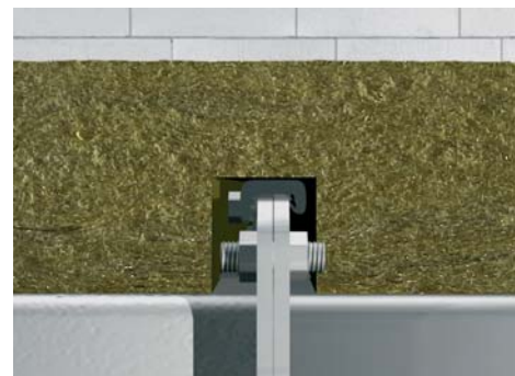
Cutting for a duct joint.
